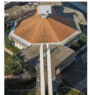
STM Church Roofing Project
